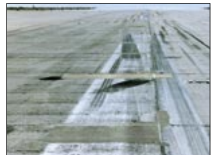
Leipzig/Halle Airport: Repairing concrete, runways and taxiways
