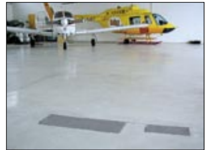
Mannheim Airport Repairing hangar floors
