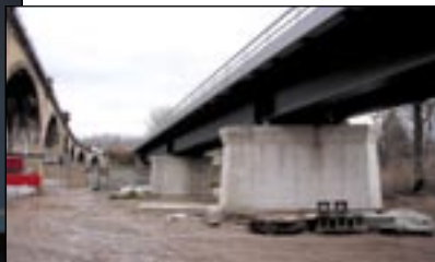
Viaduct construction in Chemnitz: Laying pillar foundations in winter
