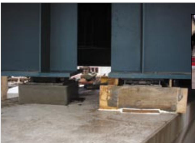
Chemnitz-Einsiedel viaduct, Blankenauer street: repairing bridge bearings
