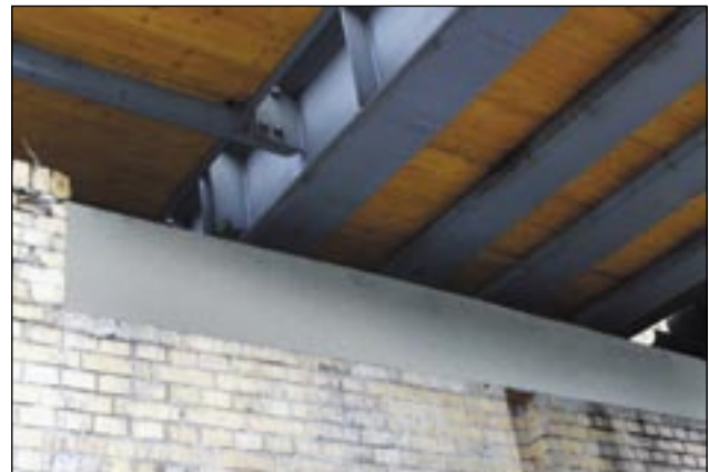
Metropolitan viaduct, Berlin, Sterndamm: repairing bridge bearings
