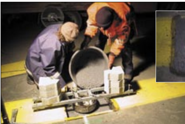
Nordrhein-Westfalen Airport: Replacing and installing embedded runway lights without air-traffic interruption
