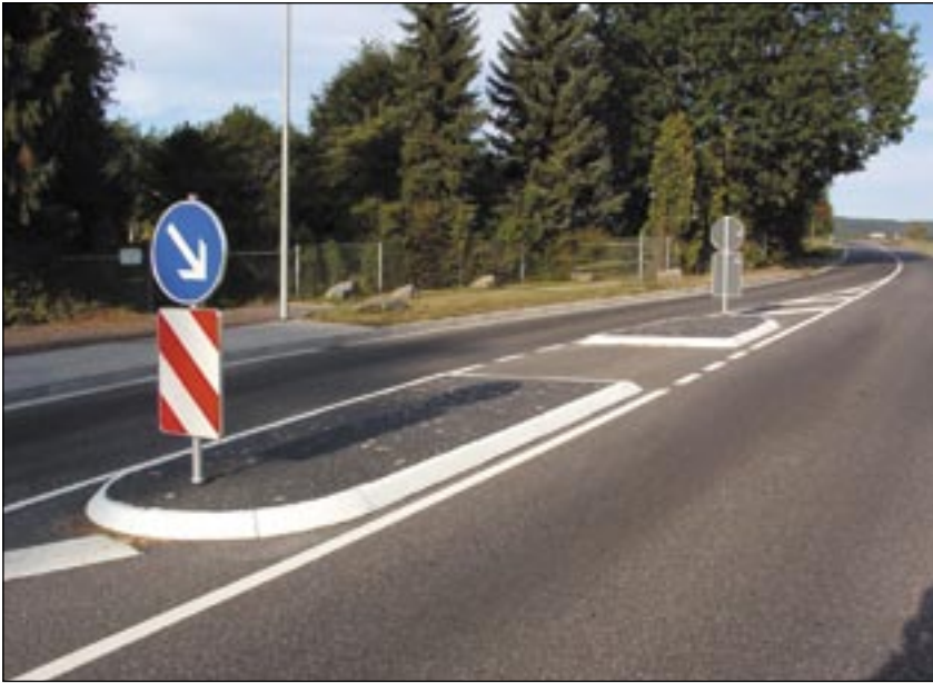
K 106 by-road, Neuwied-Niederbieber: Kerb of a traffic island stuck to the asphalt with SILIKAL® Mortar R 17
