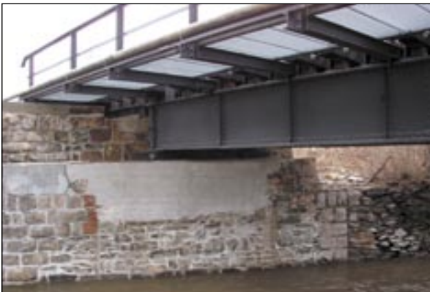
Chemnitz-Einsiedel viaduct, Blankenauer street: repairing bridge bearings
