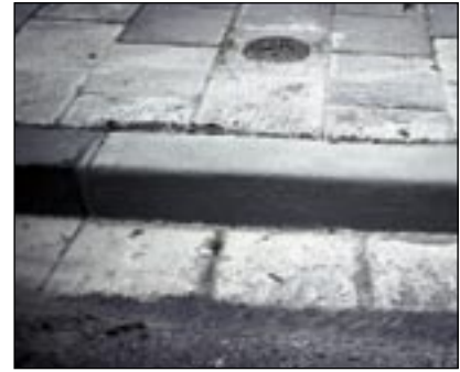
Repairing the kerbs with SILIKAL® Mortar R 17
