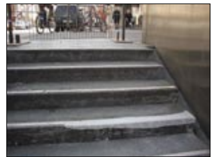
Metro station stairs in Venloer street, Cologne: repairing the steps
