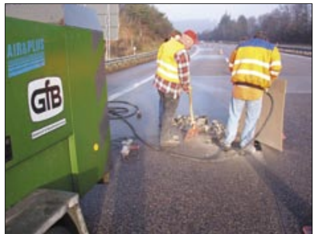
A3 Motorway, Neustadt/Wied: Improving the road surface
