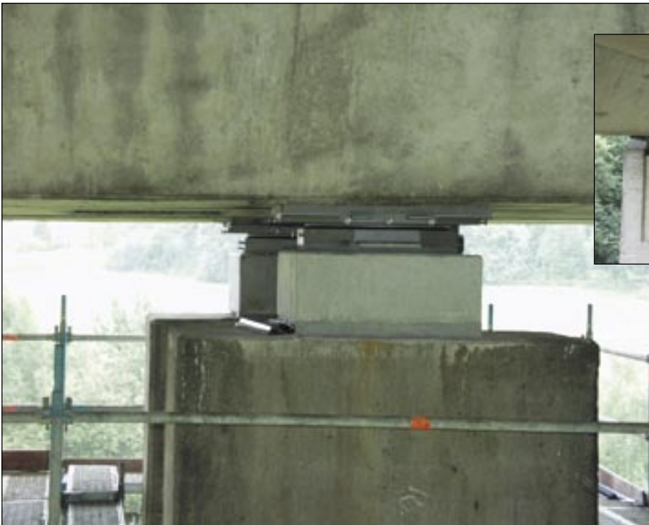
A7 motorway bridge, Uttrichshausen: Repairing bridge bearings
