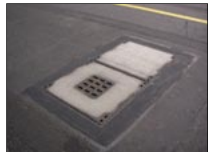
Nordrhein-Westfalen Airport: Sealing cable ducts with asphalt-coloured SILIKAL® Mortar R 17
